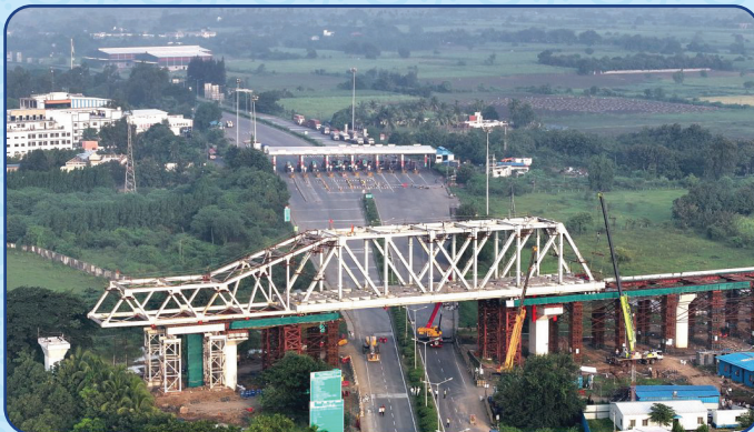
First Steel Bridge of 70 metres length
