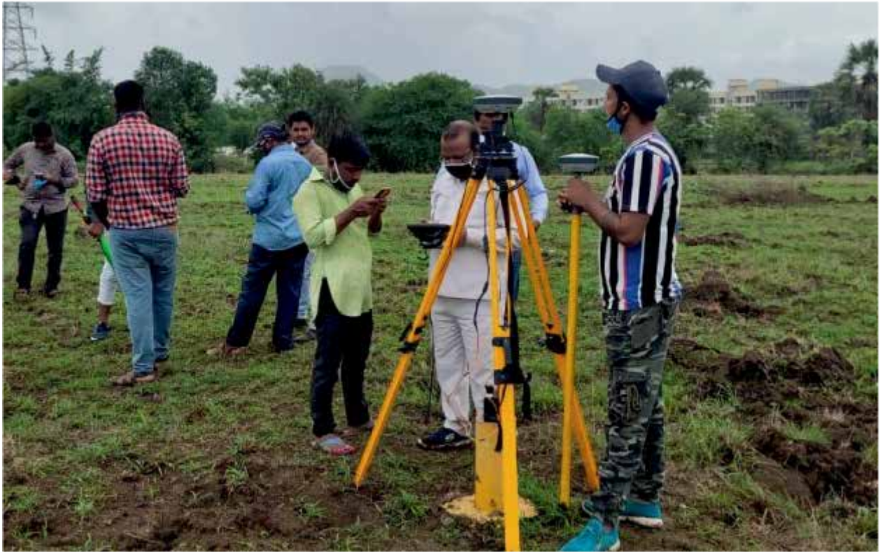
Joint Measurement Survey at Boisar HSR Station site
