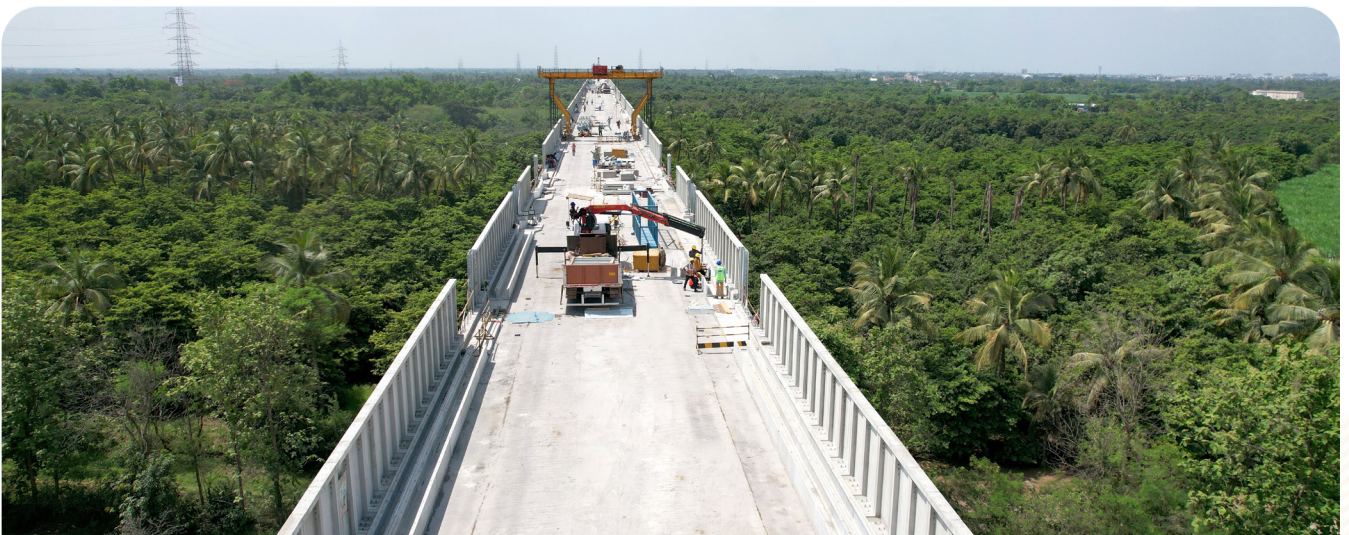
Noise barriers installation on MAHSR viaduct at a location near Surat, Gujarat
