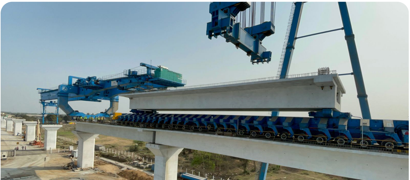
Girder Transporter Feeding Full Span Box Girder to Launching Gantry for Launching the Girder
