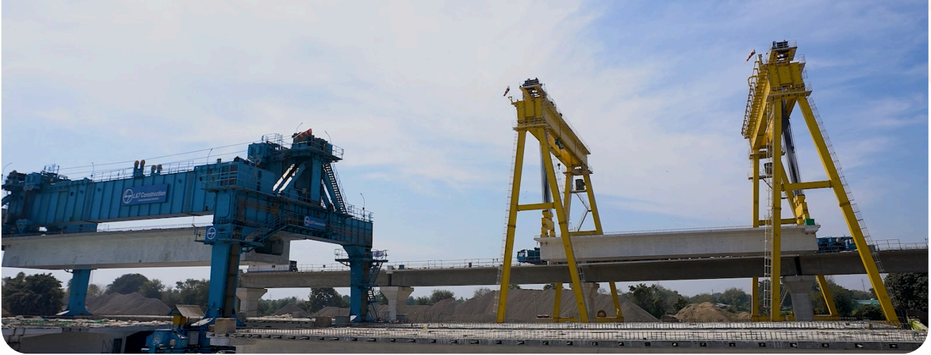
A Bridge Gantry and Straddle Carrier in action at one of the casting yards in Gujarat
