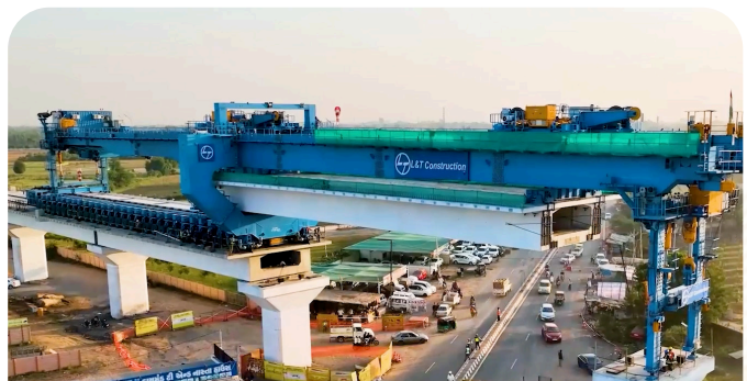
Full Span Box Girders are helpful in crossing rail/road with minimum block time
