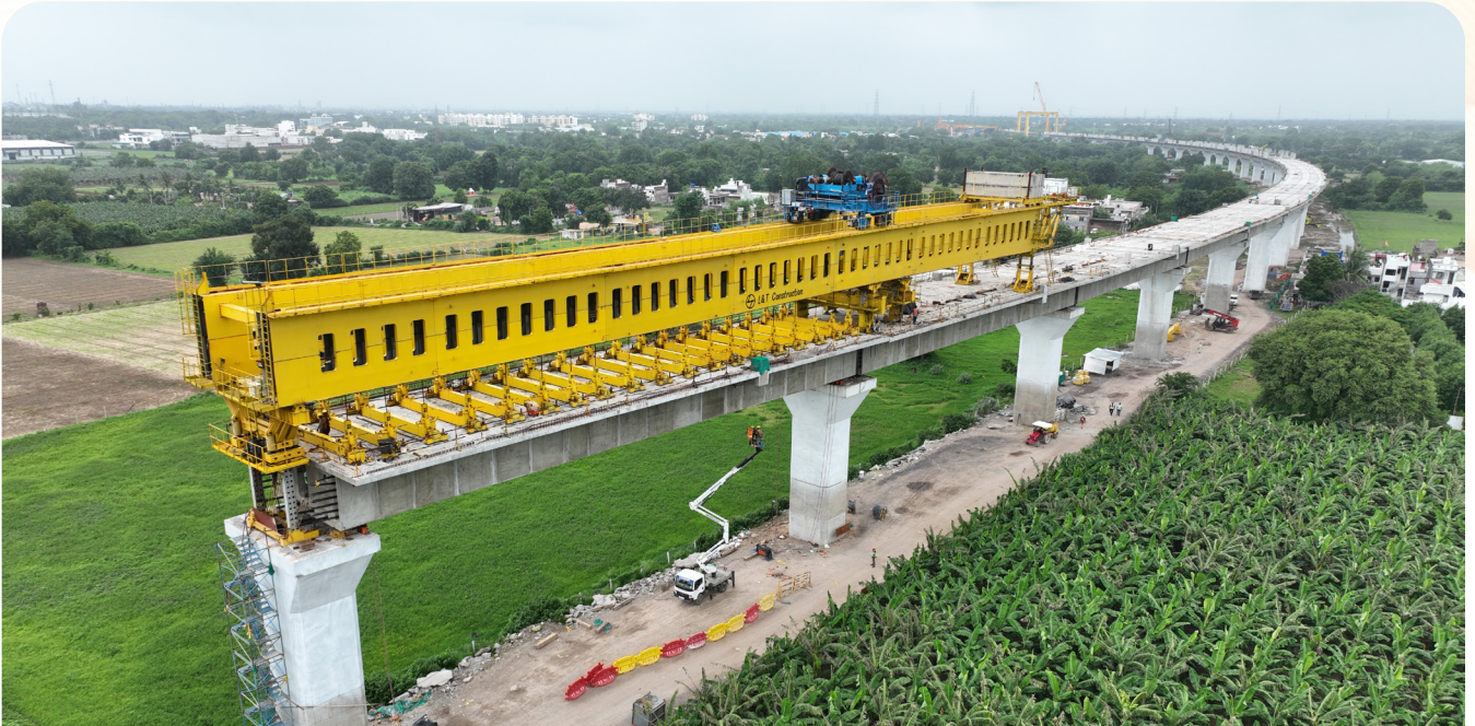
MAHSR viaduct construction using Segment by Segment (SBS) method
