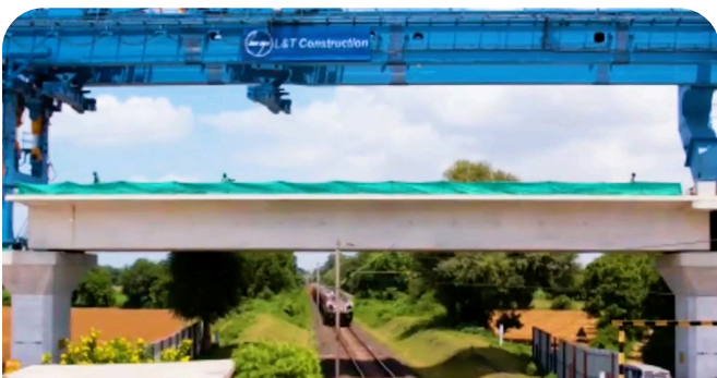
Full Span Box Girders are helpful in crossing rail/road with minimum block time
