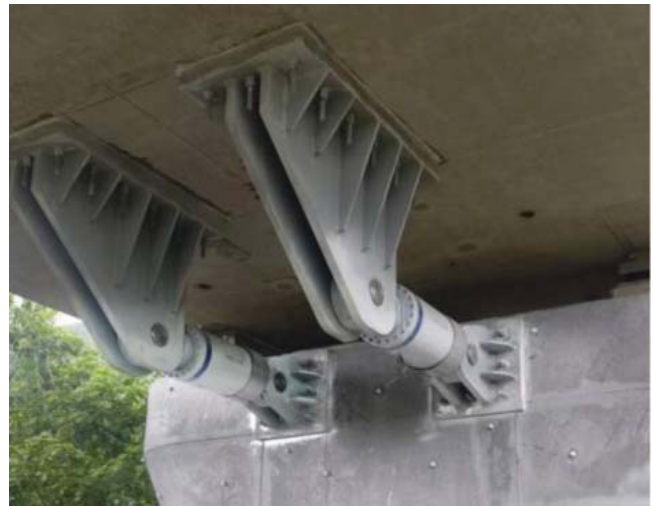
Fig. 15: Shock Transmission Unit (STU)
