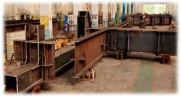
Test fabrication of end cross beam, including assembly
