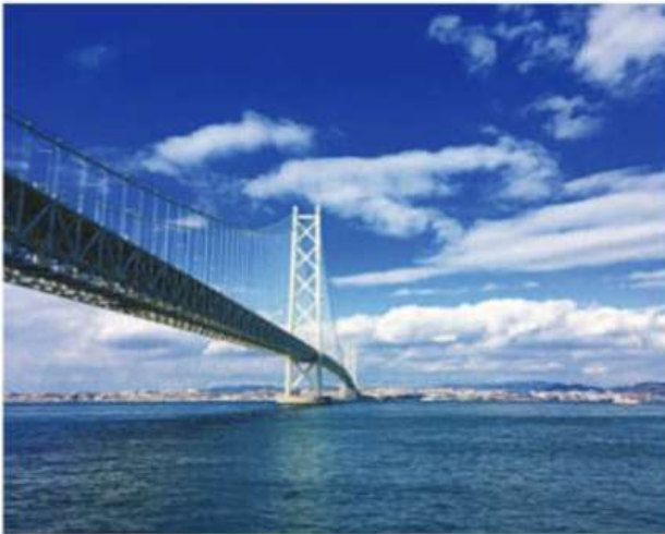
Akashi bridge, Japan
