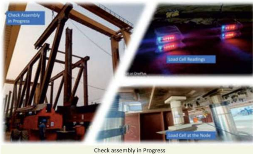
Check assembly in Progress
