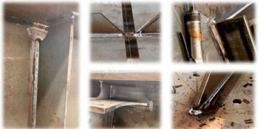
Weld Finishes, Japan
