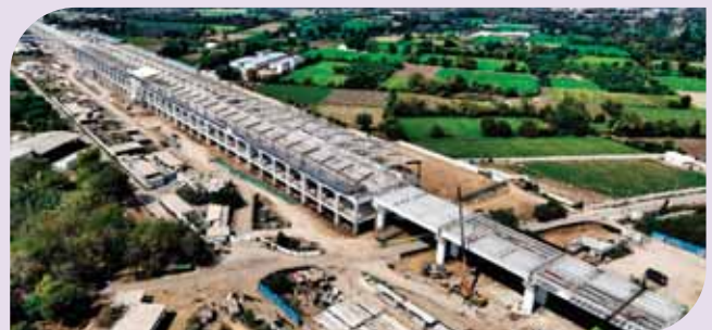
Under Construction Anand Bullet train station
