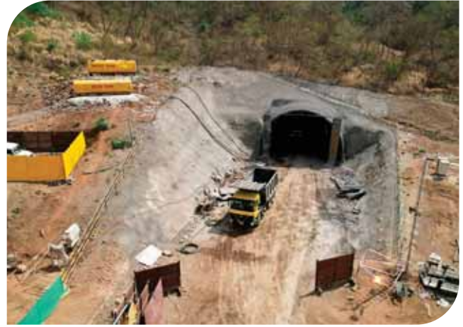
Work in progress for India's First Undersea Rail Tunnel in Maharashtra
