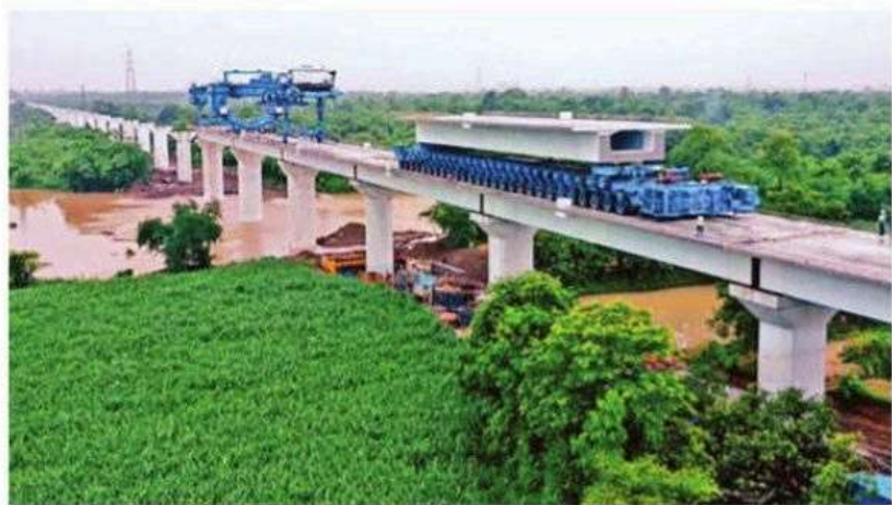
The bridge over Kolak river in Valsad district is 160 metres long
