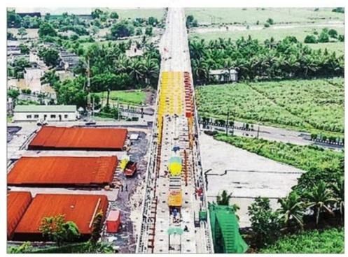
has started on this portion. The railway track slabs are ready for approximately 70km. The contract for the entire segment from Ahmedabad to Vapi, including track laying, has been awarded. As soon as the track bed is ready, the work for track laying will begin.
