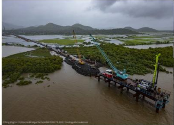
Setting up for viaduct bridge for Mumbai (CH 13.00) to Ahmedabad
