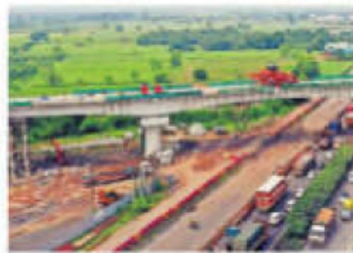
**Bridge comprises 72 precast segments with four spans.**
