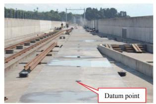
Figure 9.7-17 Reinforced Concrete Track Bed at Turnout
