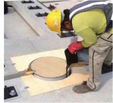
Figure 9.7-67 Injection of Urethane Resin around the Concrete Projection
