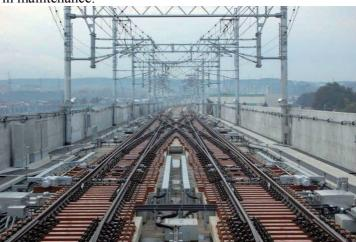
Figure 9.7-14 Synthetic Sleeper Ballast-less Track
