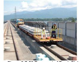
Figure 9.7-59 Transport of Track Slabs
