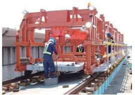
Figure 9.7-63 Laying of Track Slabs
