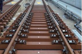
Figure 9.7-32 Simplified Shinkansen Type Expansion Joint
