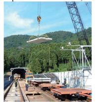
Figure 9.7-58 Loading the Train with Track Slabs
