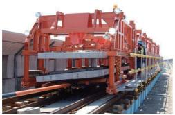
Figure 9.7-62 Lifting of Track Slabs
