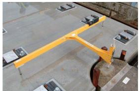
Figure 9.7-64 Adjusting of Track Slabs
