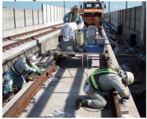
Figure 9.7-72 Insertion of Variable Pads
