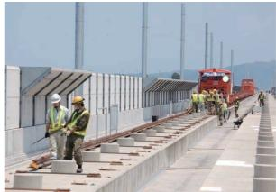
Figure 9.7-57 Rail Sliding-out Operation
