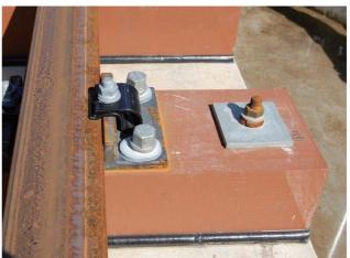
Figure 9.7-90 Fastening of Sleeper
