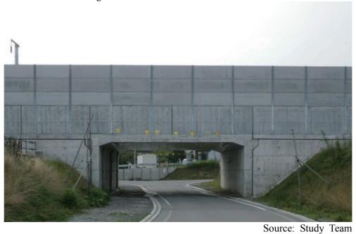
Figure 9.2-19 An Image of Box Culvert RUB
