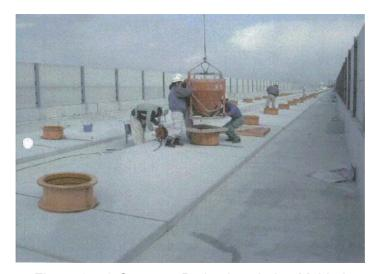
Figure 9.7-9 Concrete Projections being Molded
