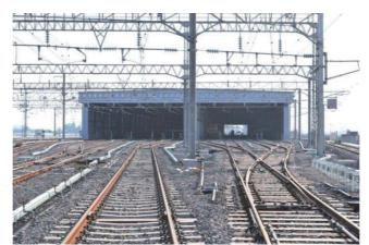
Figure 9.7-19 Ballast Tracks at Rolling Stock Bases
