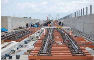
Figure 9.7-88 Fabrication of Turnout
