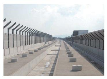
Figure 9.7-10 Completed Reinforced Concrete Track Bed
