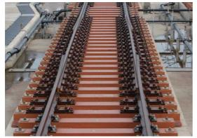
Figure 9.7-31 Shinkansen Type Expansion Joint
