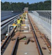
Figure 9.7-60 Expansion of Track-gauge
