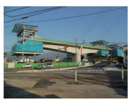
Figure 9.4-5 RUB (Continuous Bridge of PC – Box Girder using Cantilever Method)
