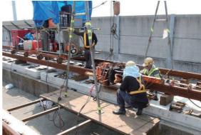
Figure 9.7-68 Relocation of Rails
