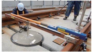
Figure 9.7-70 Adjusting of Rails
