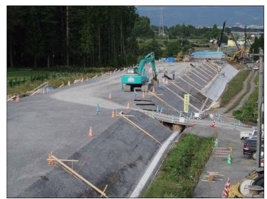
Figure 9.2-12 Japanese Experience of the Reinforced Embankment Structure
