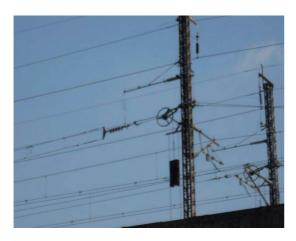
Figure 9.10-24 Pulley type ATD
