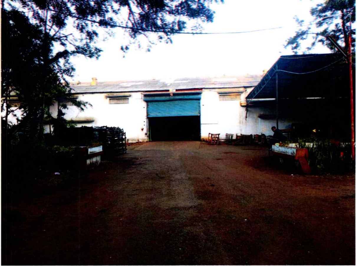
Main Industrial shed
