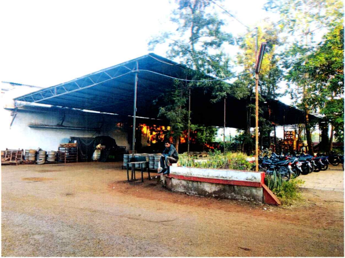
A.C sheet front Roof Shed
